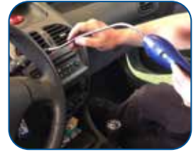
Leak in the evaporator.
