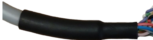
Correctly applied heat-shrink at the cable jacket end
